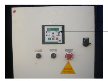
Engine controller. AGC 242 will give start input to engine controller for starting the DG
