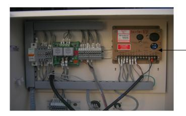
Analouge output from AGC 242 connected to GAC Governing card for Speed Regulation.
