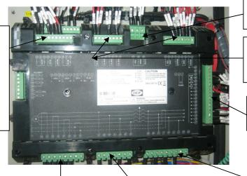
Terminal for Crank/Run and Emergency Stop.
